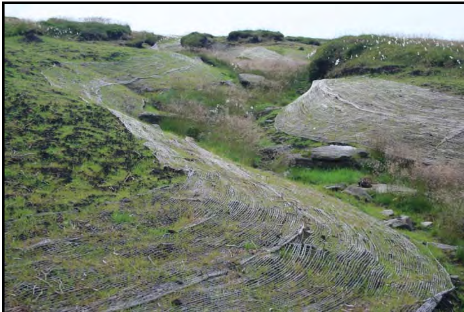
Photograph 16 Slope Stabilisation Using Geojute Matting (note the re-vegetation following addition of lime, grass and heather seed, fertiliser and heather brash)
