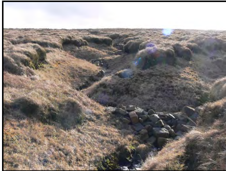
Photograph 7 Recent Gully Blocking Work with Local Stone Blindstones Moss, Ashway Gap
