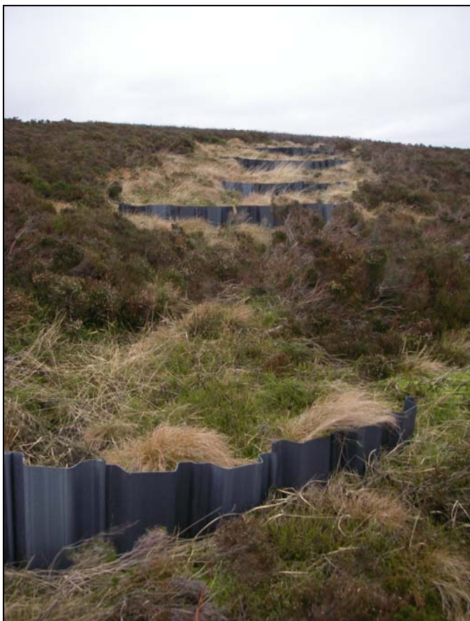
Photograph 1 Grip Blocks Made from Plastic Sheet Piling
