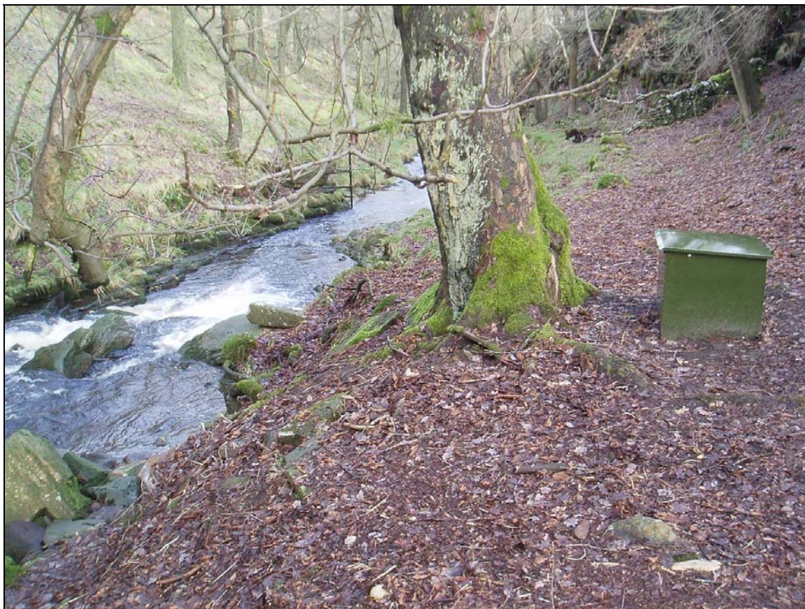
Photograph 1 Secure, Weather-Proof Equipment Housing – Upper Goyt Stream Monitoring Site (Note the Black Stilling Well in the Background – Left Bank of River)
