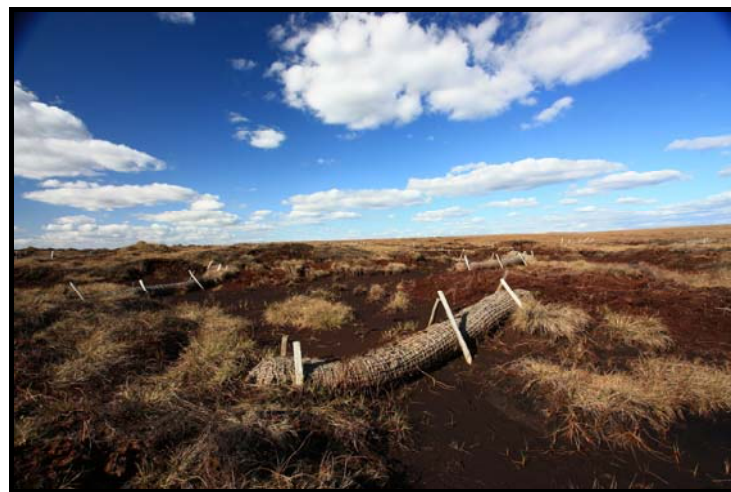
Photograph 4 The Bare Peat Pans on the Ashway Gap Monitoring Site Prior to Restoration, also Showing the Installation of the Coir Rolls
