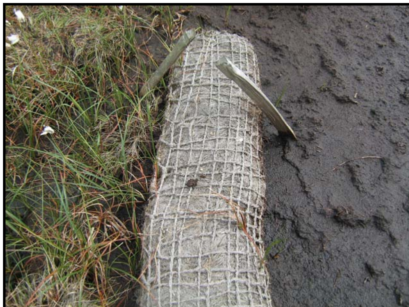
Photograph 17 Coir Roll on Ashway Gap Showing Peat Accumulating and Vegetation Colonising Behind the Coir Roll (Note the uneven surface of the exposed bare peat indicating the surface 'downstream' of the coir roll is still highly mobile and vegetation establishment is likely to be compromised)
