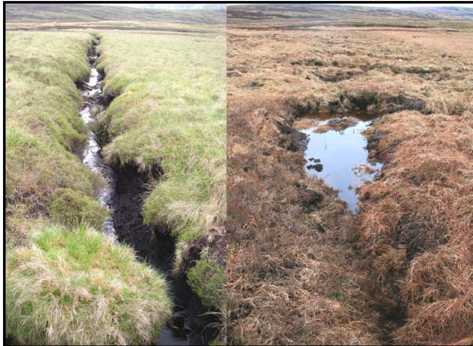
Photo 3 Brennand Brown Syke Sub-Catchment Before (May 2007- left) and After (February 2009 - right) Major Grip Blocking Work was Completed
