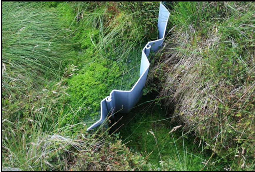
Photo 4 A Blocked Grip in the Whitendale Catchment where Vegetation Succession is Beginning to Fill in the Channel. In this Case, Sphagnum fallax is Building up in the Old Grip
