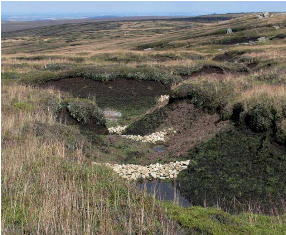
Figure 7. Low dams of stones holding water in deep gullies.
