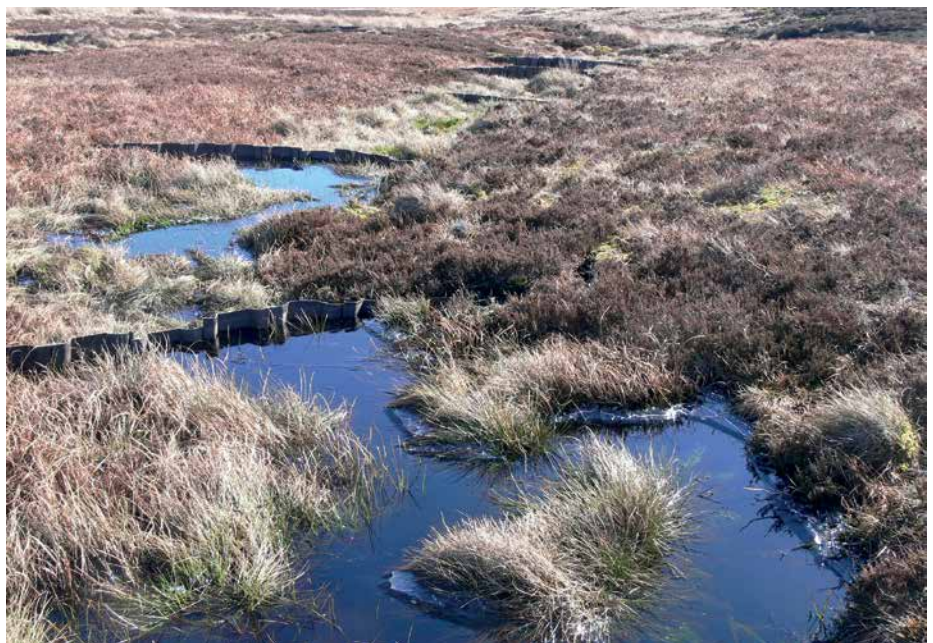
Figure 3. Plastic dams in a gully, raising water tables in the peat
