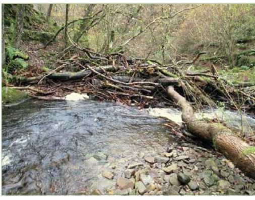
Woody debris dam constructed on River Aller
